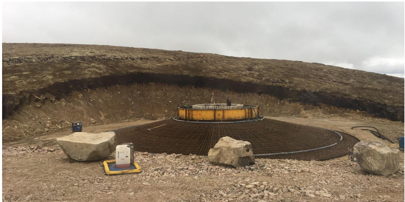
Wind turbine foundation
